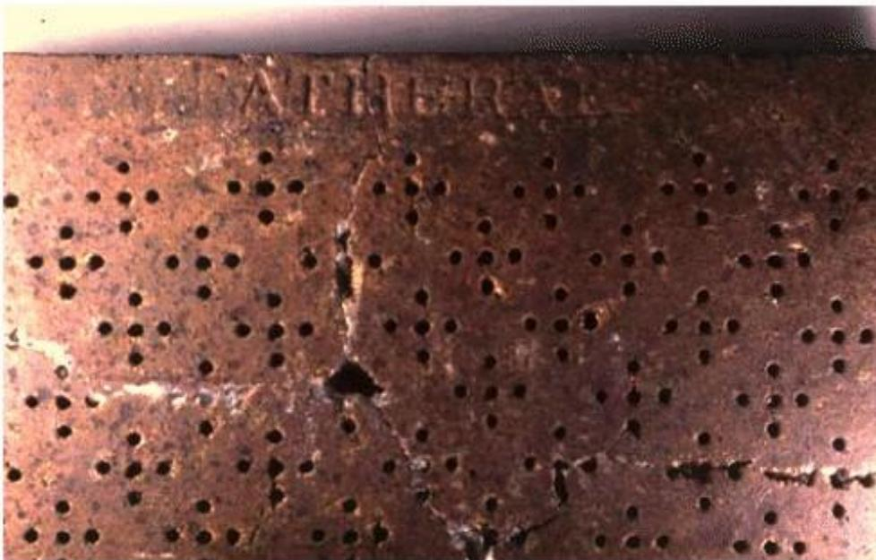
*A late Buckley tile with diamond-shaped cells and five perforations, stamped on the face with CATHERALL; from Melin Tyddyn Du, Maentwrog, Gwynedd.*
